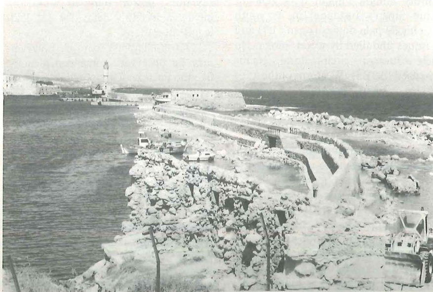
Mudjacking the crumbling foundations of the Venetian mole
