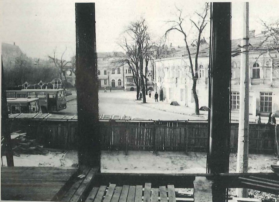
The house was in such a ruined state that it had to be demolished and rebuilt from scratch.
