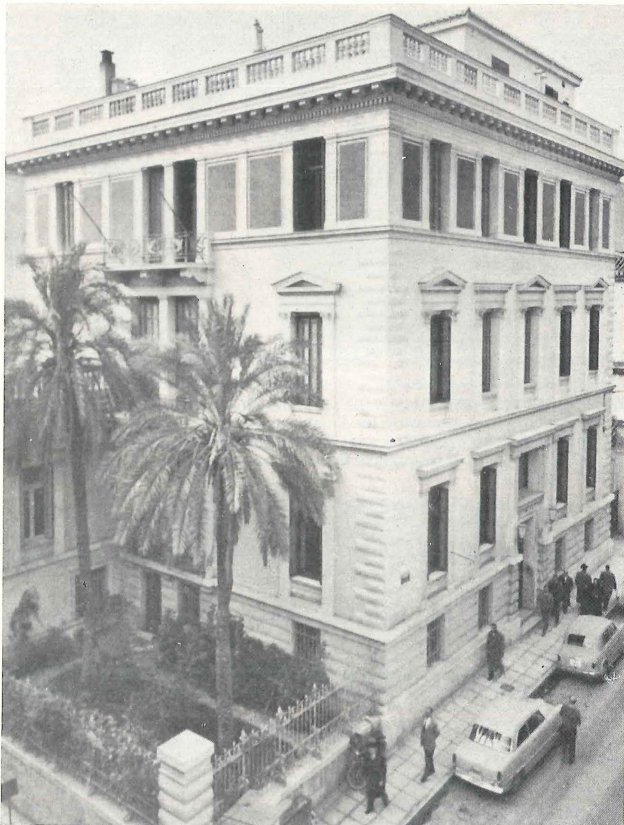
The German Archaeological Institute on the corner of Fidiou and Harilaou Trikoupi was built in 1897 according to designs commissioned by Heinrich Schliemann from Ernst Ziller, the Dresden-born architect who built many of Athens' finest neoclassical buildings
