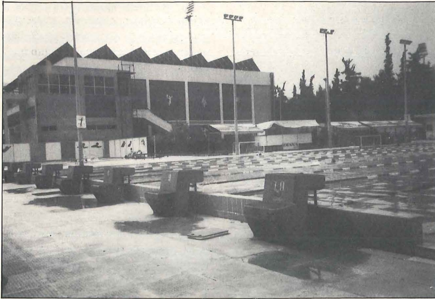
Illisia pool and sports hall
