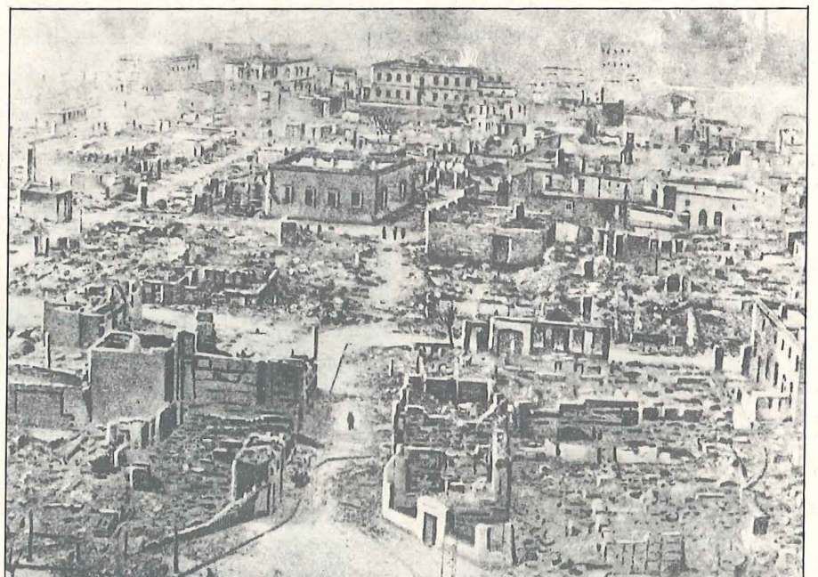
Little survived the blaze, which devastated some 9500 buildings
