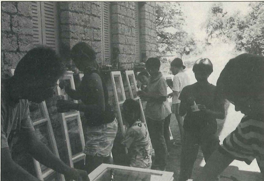
Painting windows at the Kapessovo school
