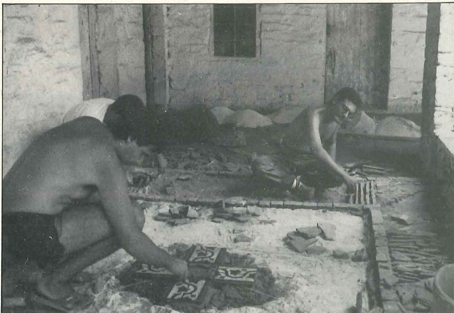
Laying traditional Byzantine floor, Trikeri
