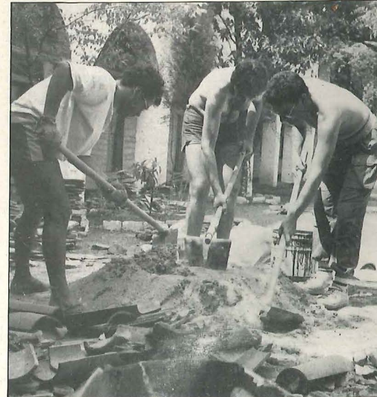
Mixing cement on the grounds of the Trikeri Monastery
