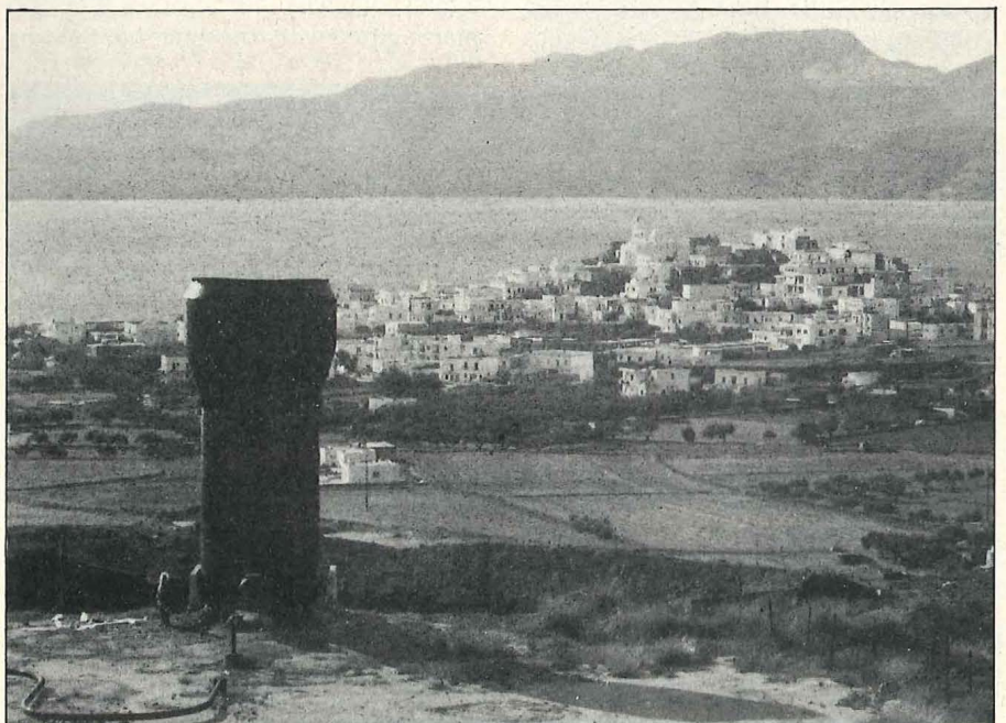
Commencement of well construction above the town of Adamas
