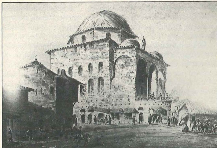
The mosque in 1832, by Skene, showing subsidence of the ground
