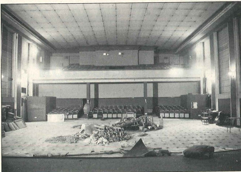
'Ideal': the Spentzos cinema being renovated
