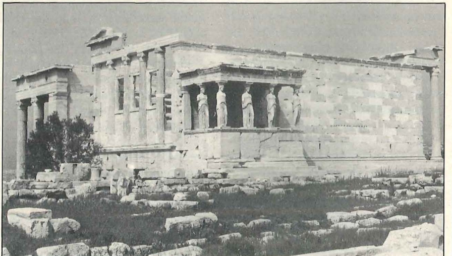
The completed restoration
