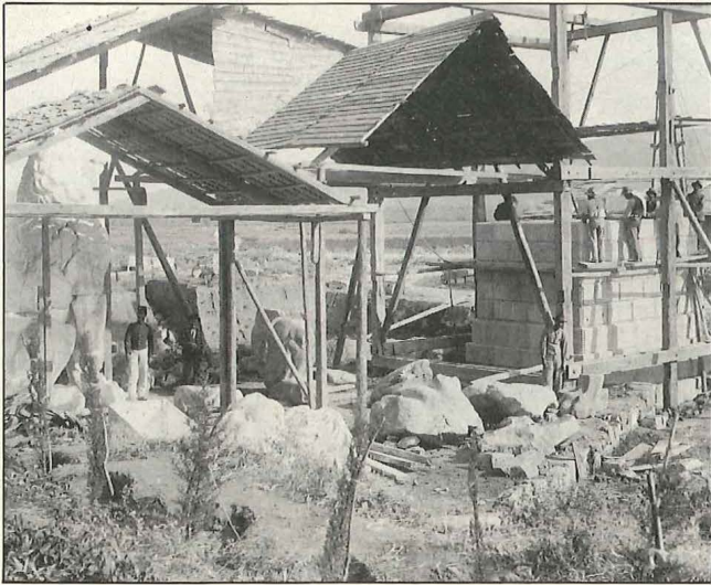
In 1902-4 the Society reassembled and restored the Lion of Chaironeia. In this 1903 photograph, the cast of the lion, now in the court of the Thebes Museum, is on the left, the pedestal on the right, and fragments of the lion itself at center. The restoration was led by sculptor Lazaros Sohos and architect N. Balanos.
