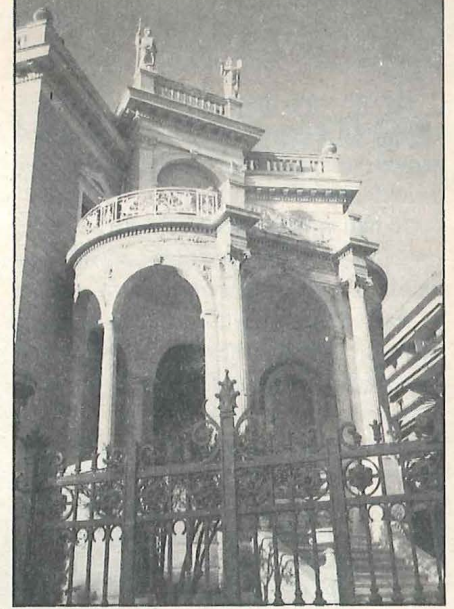
The corner staircase
