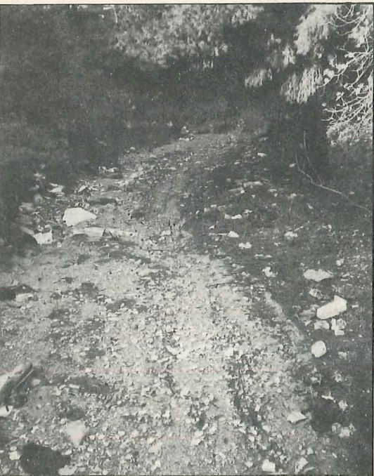
The rubbish-strewn bed of the Skripa at Frangoklissia
