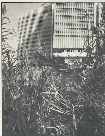
The Sappho streambed beneath the OTE building at Maroussi
