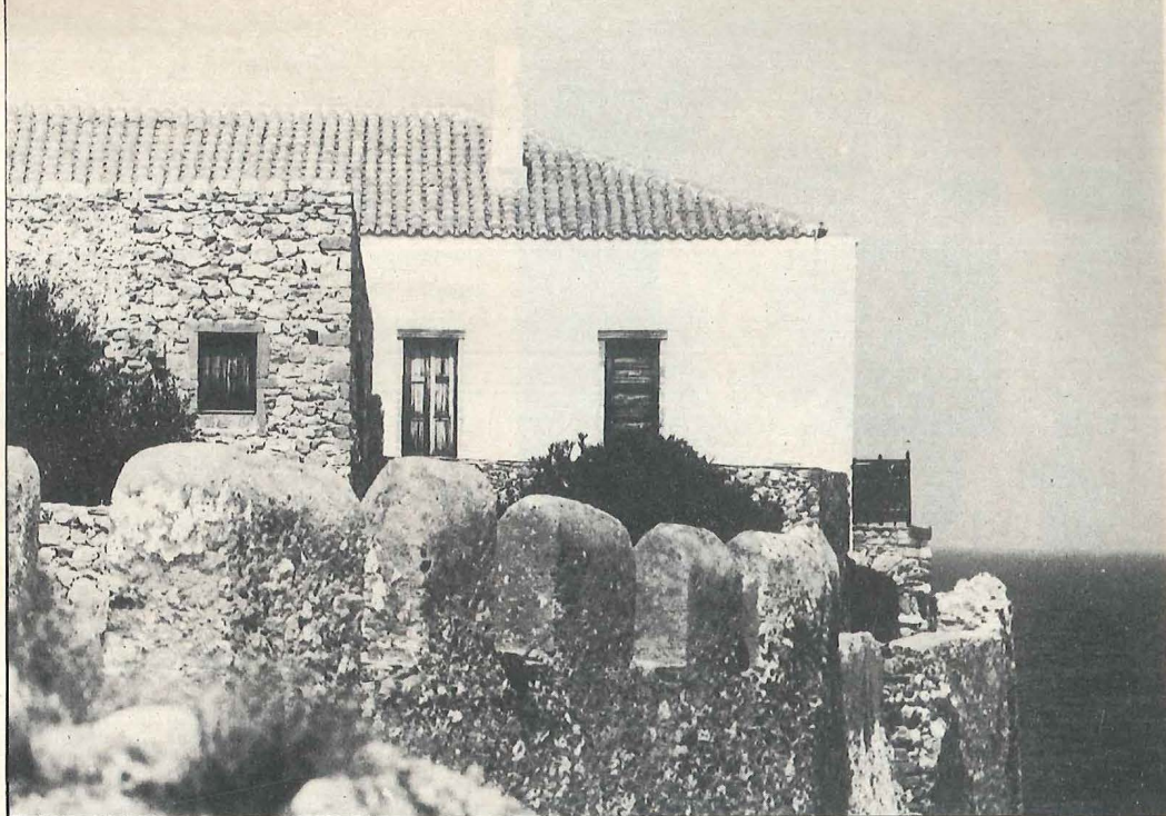
The first house remodeled by the Kalligas', with a balcony built upon medieval battlements
