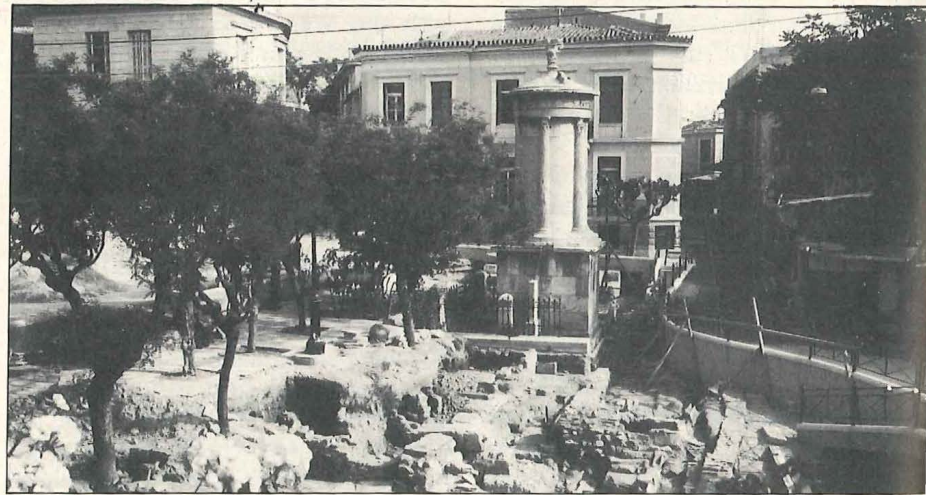
The Lysicrates monument today: part of the 'ark-park' system
