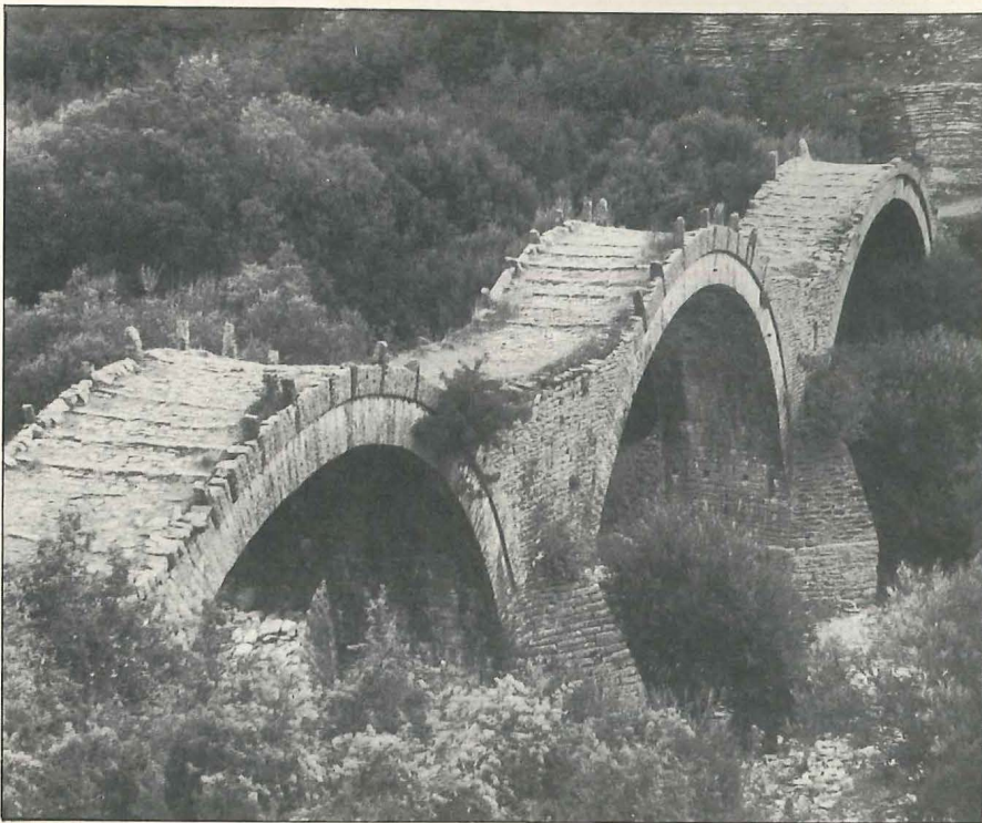
The Plakida bridge at Kipi
