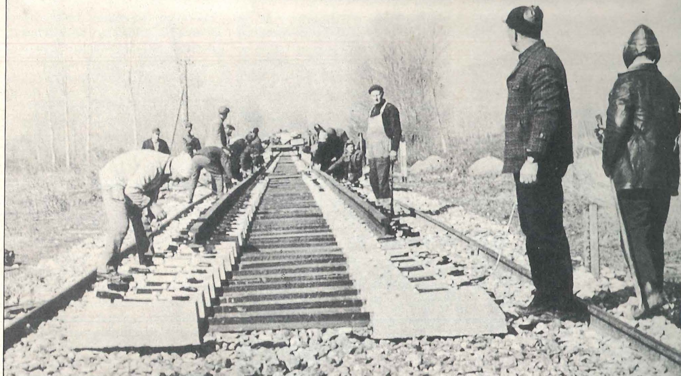
Laying a new track
