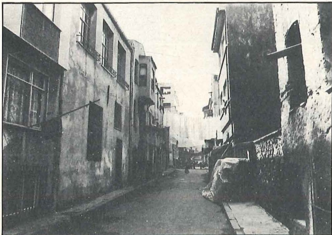
A typical street in the old city
