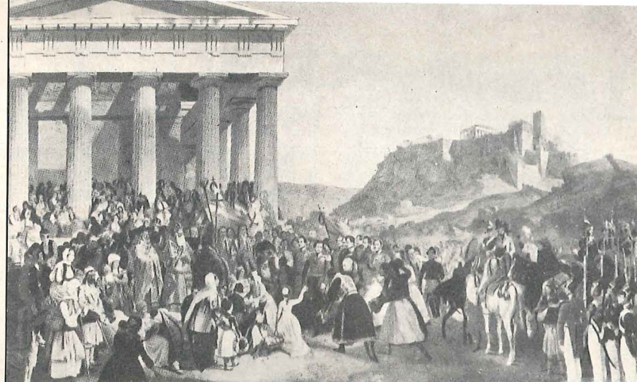
On 1 December 1834, King Otto dismounted at the Thission (then the Church of St. George) where a doxology was sung and the proclamation read officially establishing Athens as the royal seat and capital. (Peter von Hess, Bavarian State Collections, Munich)
