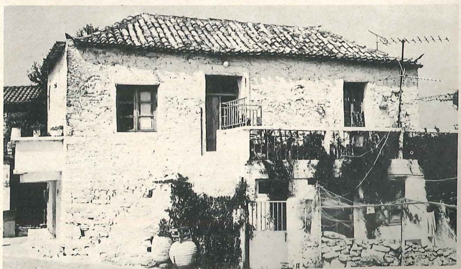
Cafeneion in main square of Skoutari; typical village house
