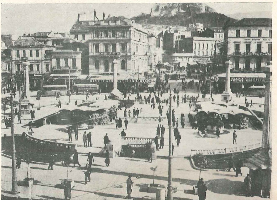
By 1932 Omonia Square had been denuded of trees. The eight columns set around the center of the Square commemorated the Muses, one Muse being omitted. The columns concealed vents rising from the underground station which served the Piraeus-Kifissia electric train. The present fountain in the Square was installed in 1961. (Benak...)
