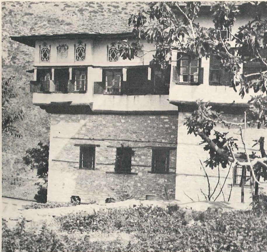
A typical Pilion house. The third floor houses the "kathistiko", a large airy living room with many windows intricately shuttered to regulate light and heat.
